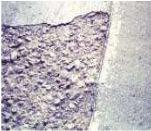
Figura 2.15 – Desgaste do pavimento (Federal Highway Administration @2016)
