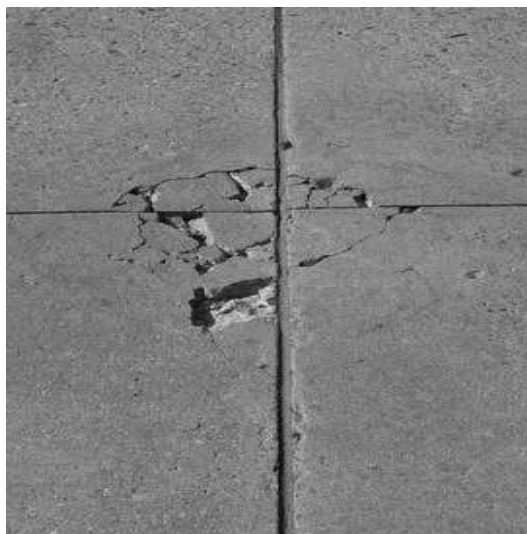
Figura 2.18 – Lasqueamento no canto (Federal Highway Administration @2016)
