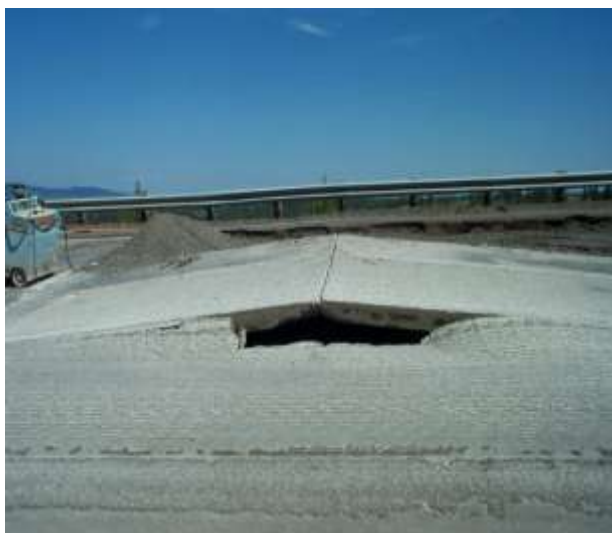
Figura 2.21 – Rebentamento (Pavement Interactive @2016)
