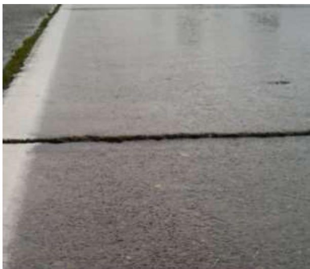
Figura 2.20 – Escalonamento (Pavement Interactive @2016)
